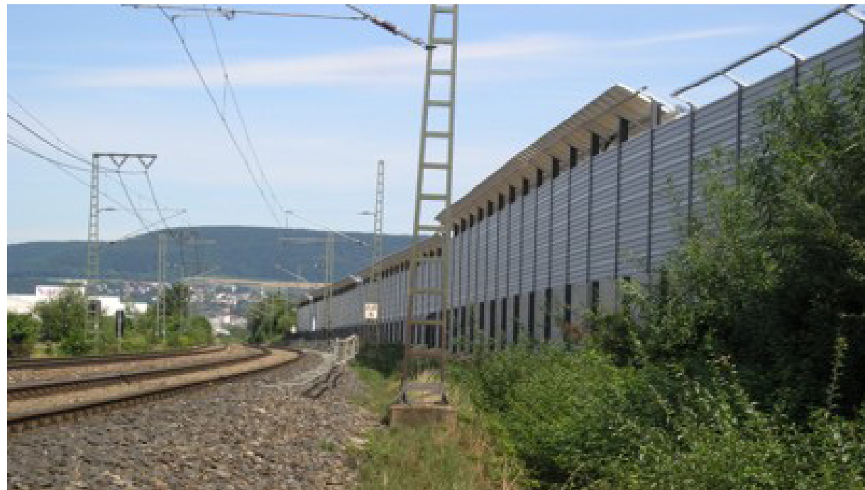
Figure 23 : Mur de contention
